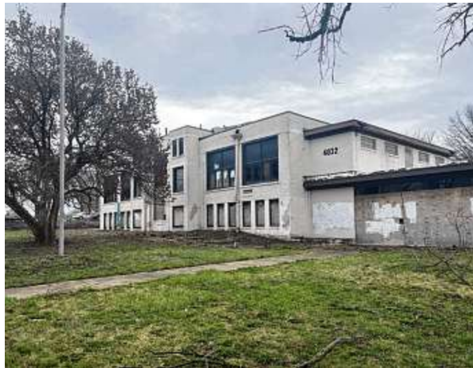
A vacant office property in Riverside that the Montgomery County Land Bank wants to demolish.
