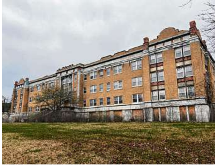
The old Fout Hall on the United Theological Seminary in Dayton, being transformed by Omega Community Development Corp.
